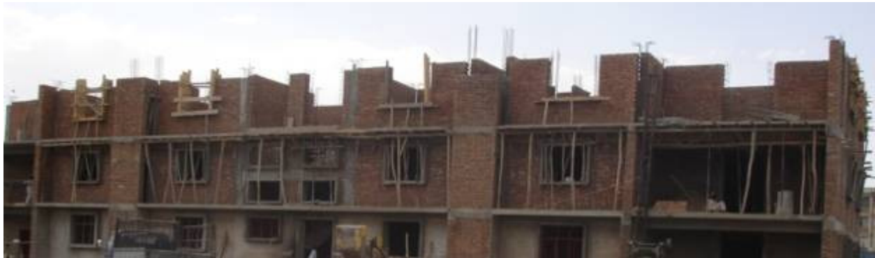
Figure 17: Female and children section under construction – Kabul August 2007
