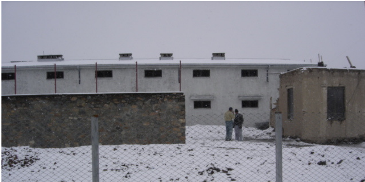
Figure 11:Gardez under construction (winter)
