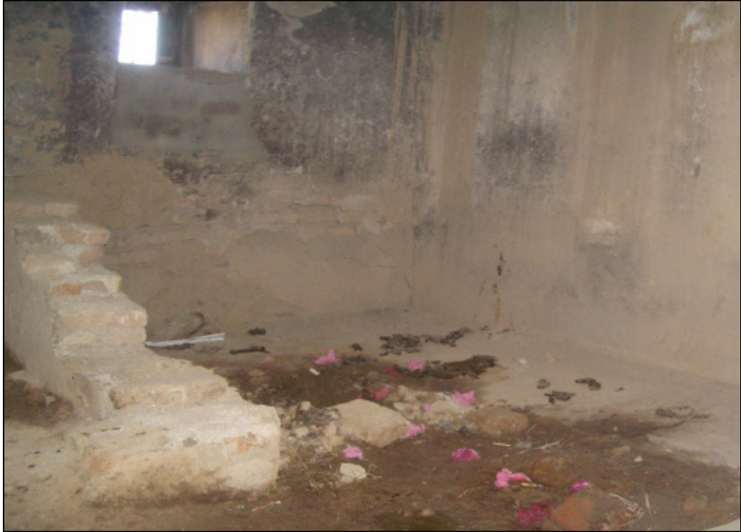
Figure 6:Gardez toilets inside the section
