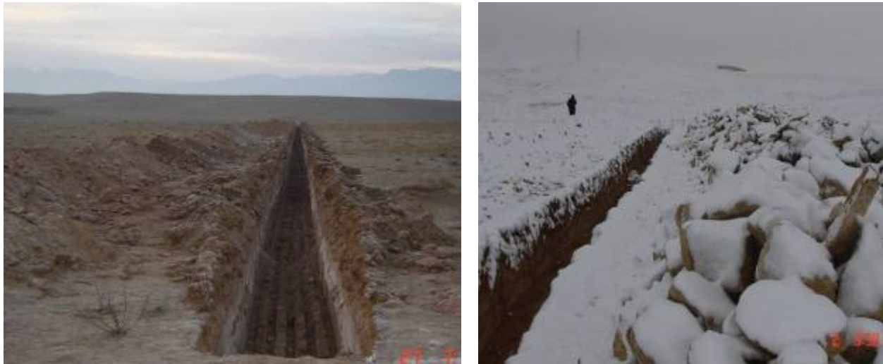
Figure 14: Mazar provincial prison new excavation for boundary wall
