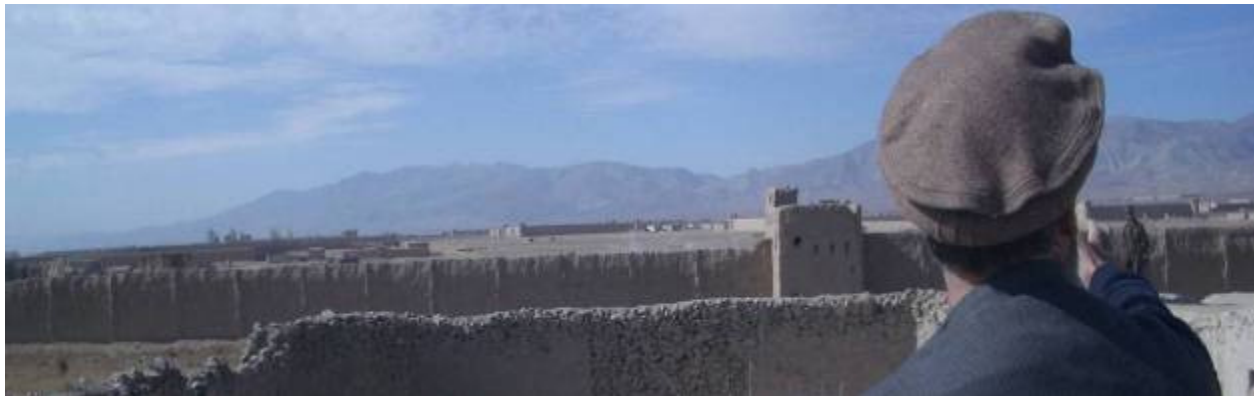
Figure 13: Gardez prison mud boundary wall prior to rehabilitation works
