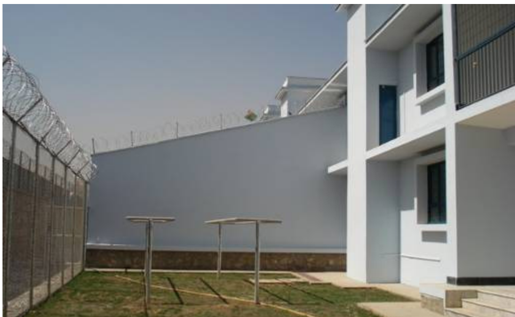
Figure 23 :Juvenile Female yard showing inner fence and visual barrier with outer fence behind
