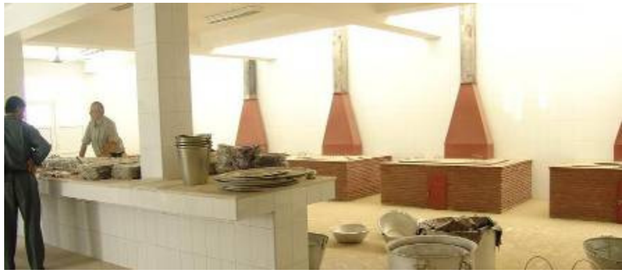
Figure 10: Prison kitchen showing open plan, central food preparation bench and fire brick stoves
