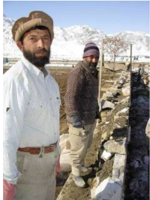
Figure 2: Masons building new wall Kabul Female & Juvenile Facility
