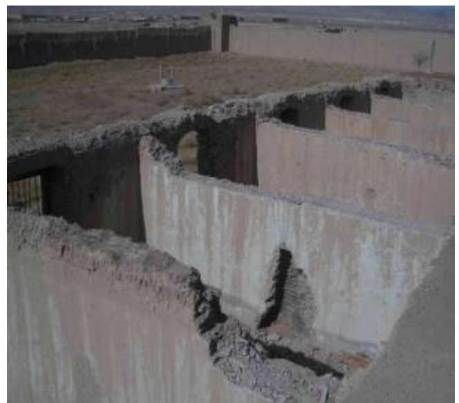
Figure 5:Gardez prison damaged wing - now repaired
