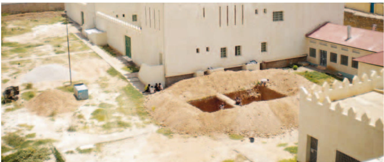
Construction of water storage tank underway at Hargeisa Prison, Somaliland
