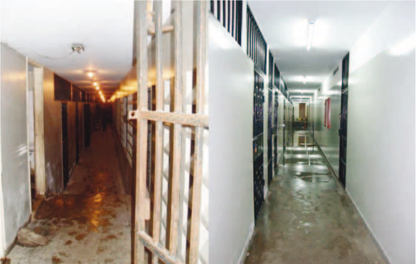
Refurbishment of Mombasa court holding cells (pictures taken March 2010 and October 2010)
