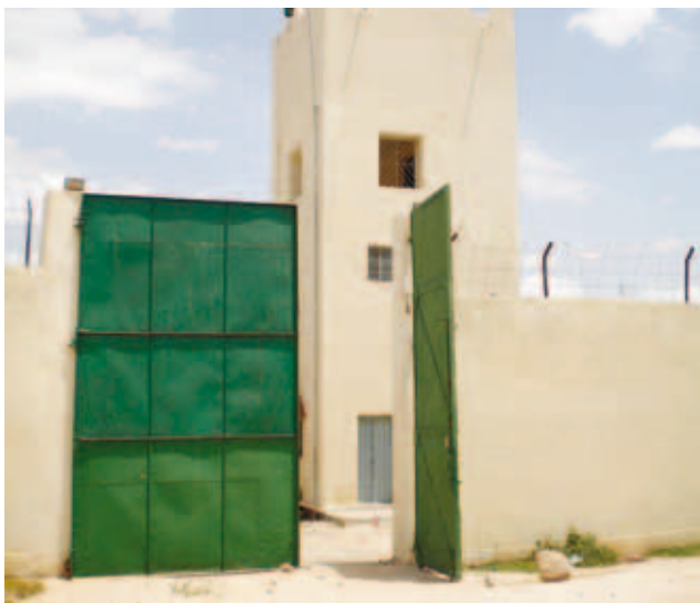
Refurbished gates and tower at Hargeisa Prison, Somaliland
