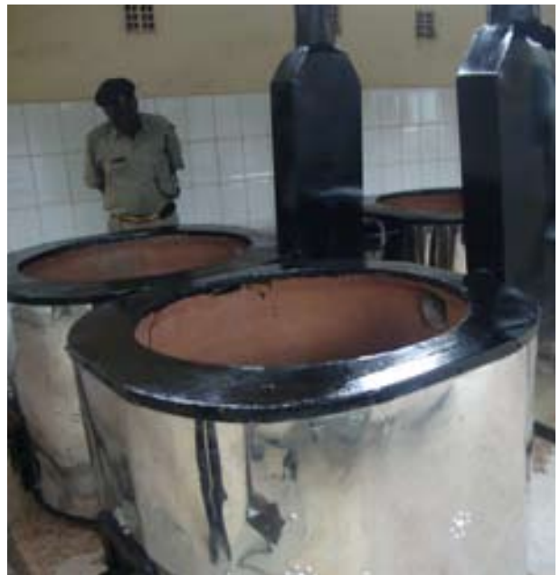
New prison kitchen built by UNODC
