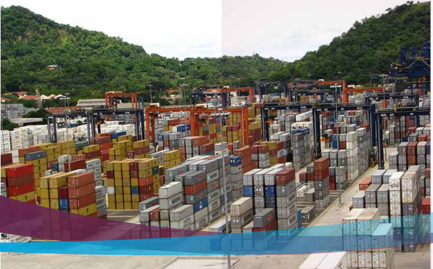
Container terminal in Panama Photo courtesy of PCU Panama
